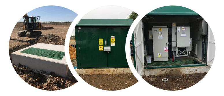
RJ Power Connections were engaged by A.C.Goatham & Son to install a 1MVA 11000/400V unit substation. This project was to provide supplies for a cold storage unit and site accommodation for a new business development. The programme of work activities were completed between March and September in 2020, with a number of key milestones across several workstreams of delivery.
