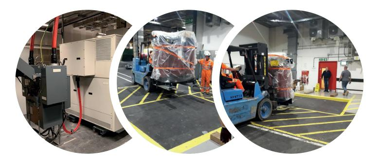
The Networks Team recently completed an extremely challenging project for CBRE as a preferred supplier within Plantation Place at 30 Fenchurch Street, installing a new Cast Resin Transformer and Housing, Ring Main Unit and associated HV cabling.
